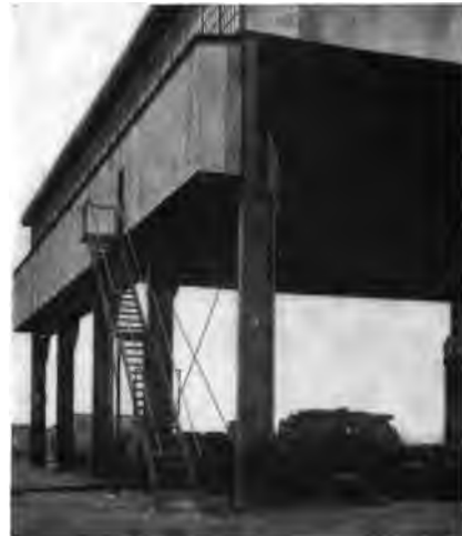
Fig. 2. Stairway Leading to Crane Runway, with Enclosed Walk on Side of Building.*
